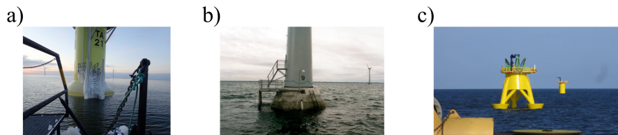
Figure 1: Three substructures with ice cones: a) GBS at Tahkoluoto [20], b) GBS of a 0.5 MW wind turbine at Tunoe Knob [17], c) jacket substructure with two ice cones at Baltic 2 [12].
